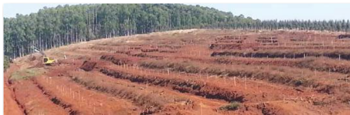
Figure 2. Appearance of the trial site during the construction of the ridges.
