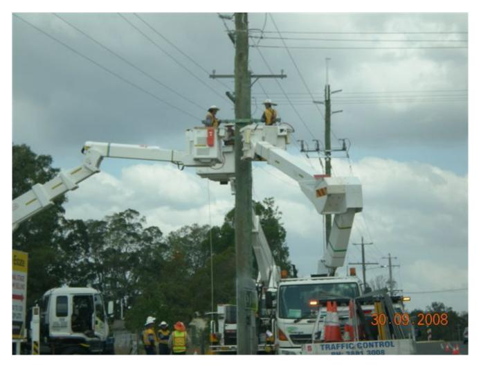
These electricity platforms are relatively sedentary once positioned. Controls are designed to prevent inadvertent movement – crush risk
