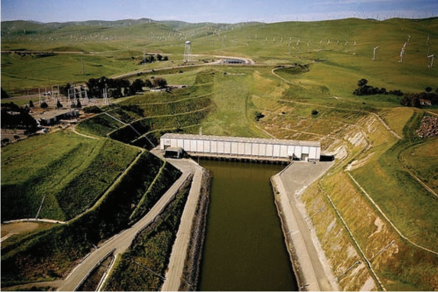
Harvey O. Banks Pumping Plant
