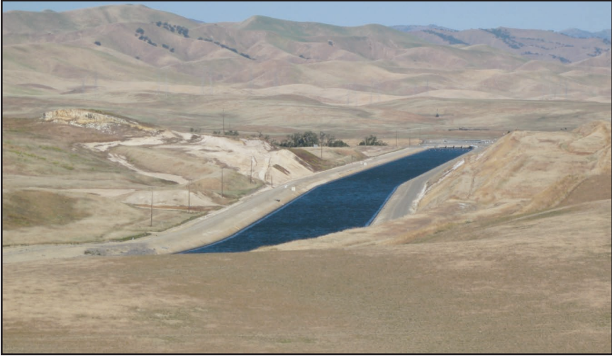
California Aqueduct through a dry Central Valley in April 2008
