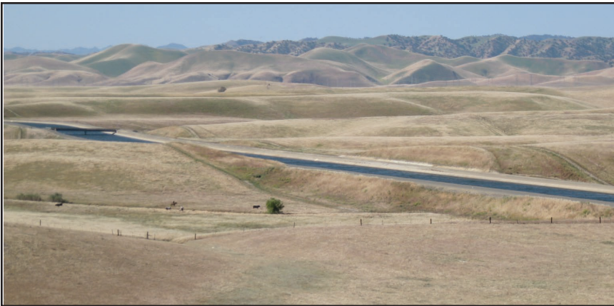
California Aqueduct through a Dry Central Valley in April 2008
