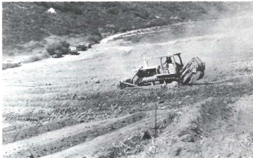
Figure 3. Tractor ripping subsoil of Bonsall sandy loam, after removal of topsoil, approximately along Line X-Y, Figure 1, preparatory to removal by scrapers. Stockpiled topsoil in foreground and beyond the ripped area.
