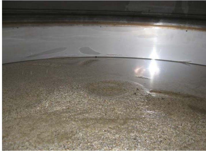
Figure 34. Lakos media bed after media cleaning
