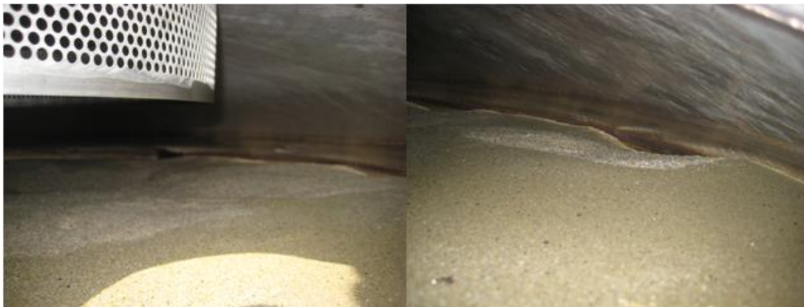
Figure 33. Flow-Guard media bed after media cleaning
