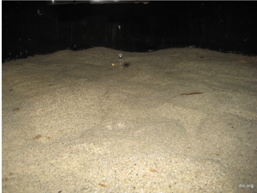
Figure 32. Arkal AGF-48" media bed after media cleaning
