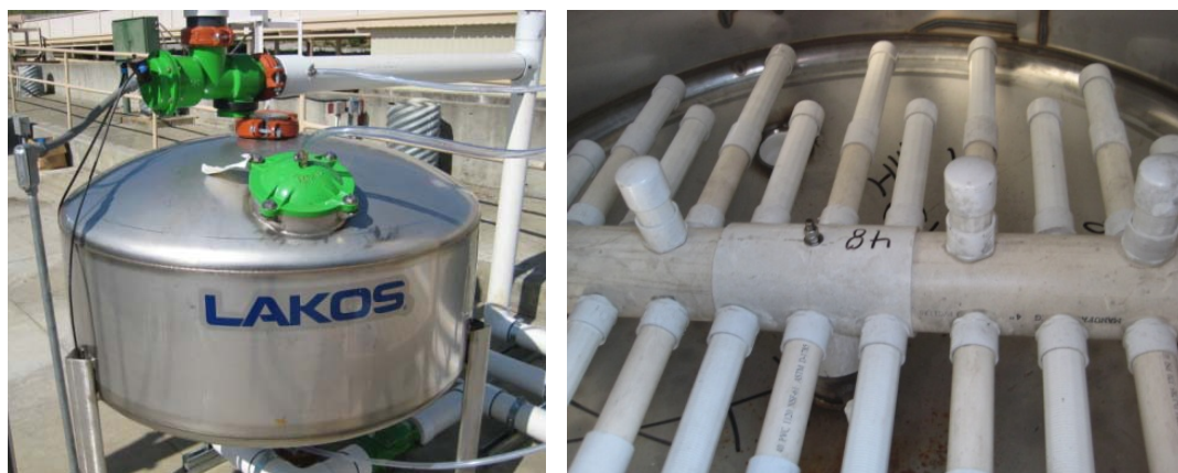
Figure 3. Lakos exterior and underdrain
