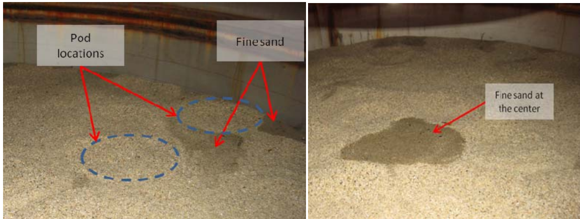
Figure 36. Waterman Dome bed after media cleaning
