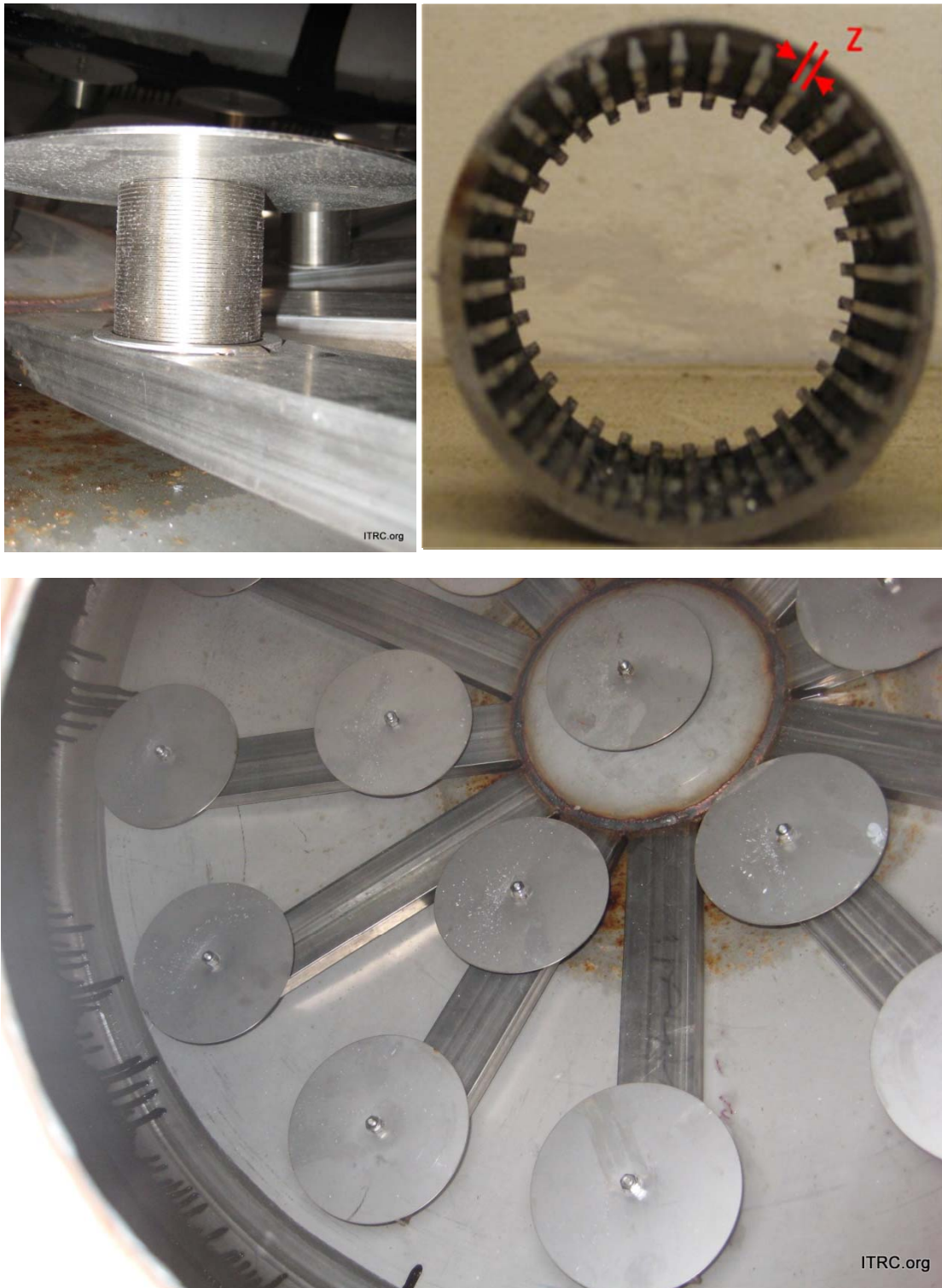
Figure 8. Flow-Guard underdrain. Pods are found under the flat stainless disks.
